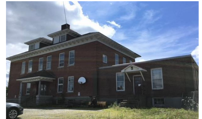
Renovation of an Historic School Building
